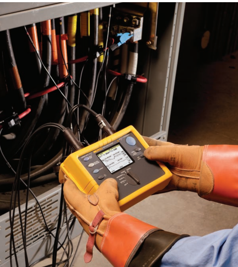
Setting up a Fluke 1735 Power Logger at the service entrance for a 30-day load study.
